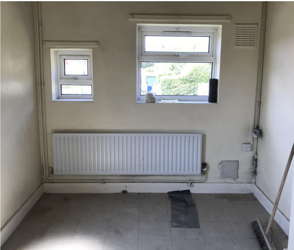
Figure 13 - internal view of flank windows serving kitchen/dining.
