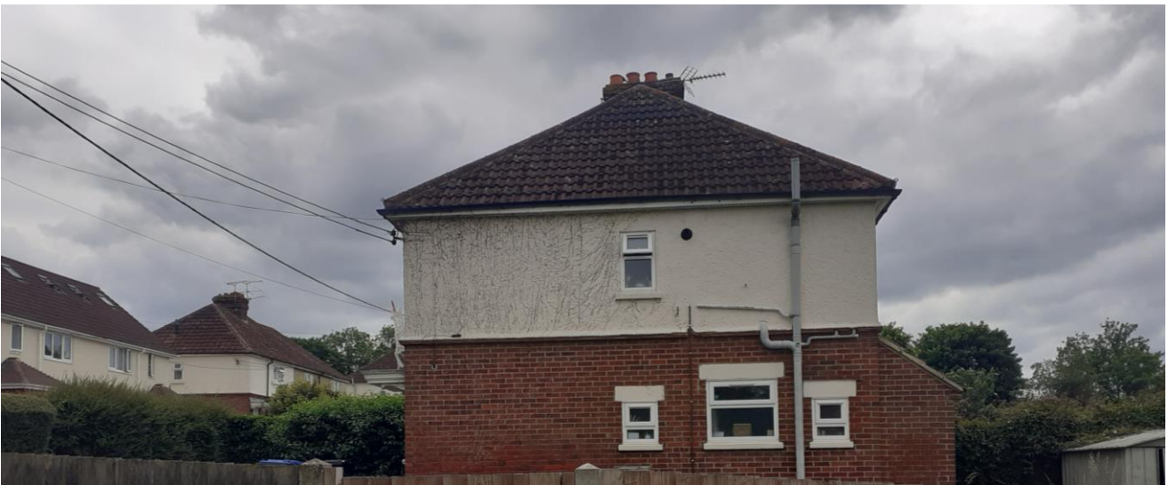
Figure 10 - Flank elevation and windows of no.8 Crownfields.
